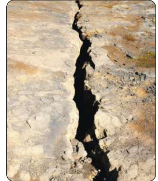
Figure (10) Earth crack
